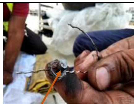
Figure-6: Upper part of the locking bolt with locking wire after removal from the wheel assembly.
