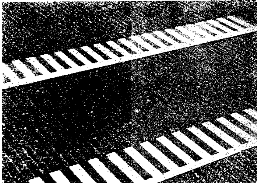
Figure 4-4. Grooving of asphalt surface (Note.- Scale shows 2.5 cm divisions)
